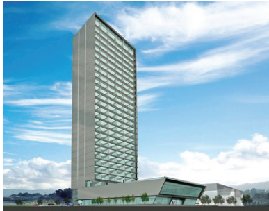
SONKAR HİLTON OTEL (Rtu, Kule)
