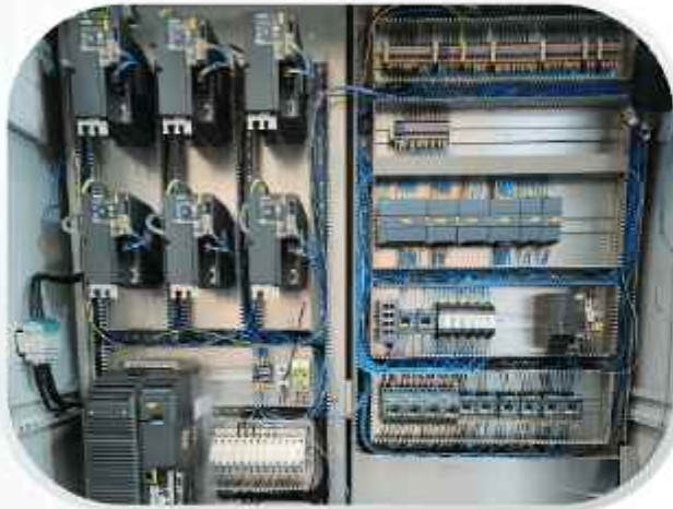
Electric Cabinet with Siemens Components
