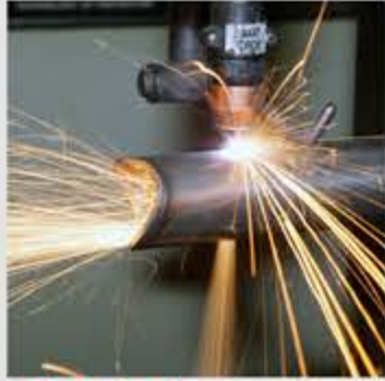
Pipe Cutting Boru kesim
