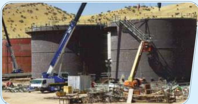
Water Tank Welding
