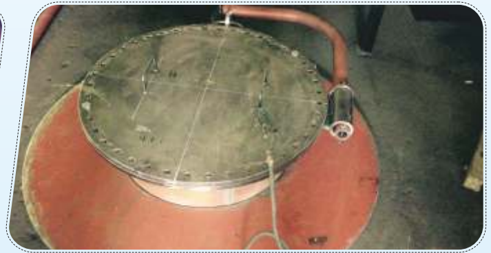
Water Tank Steel Manholes
