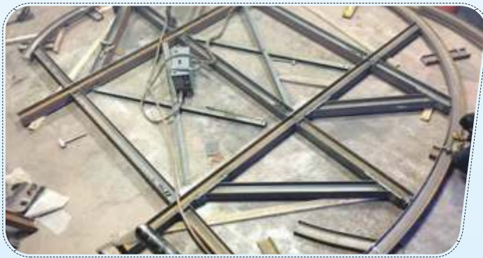
Steel Bended Tunnel Mould Manufacturing
