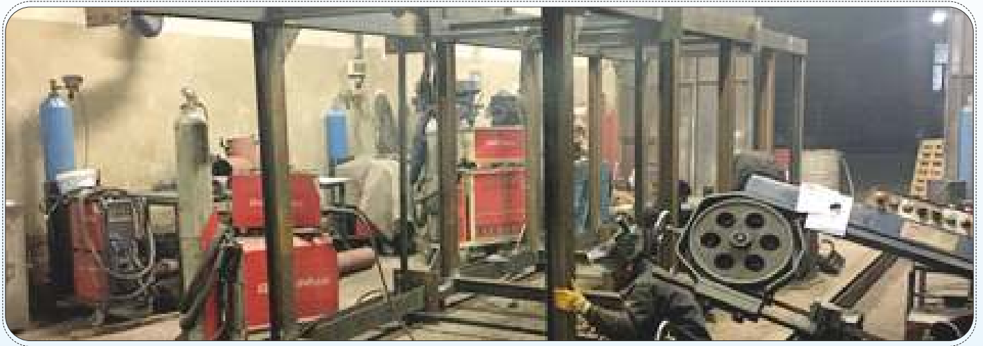
Tunnel Elevator Steel Foundation
