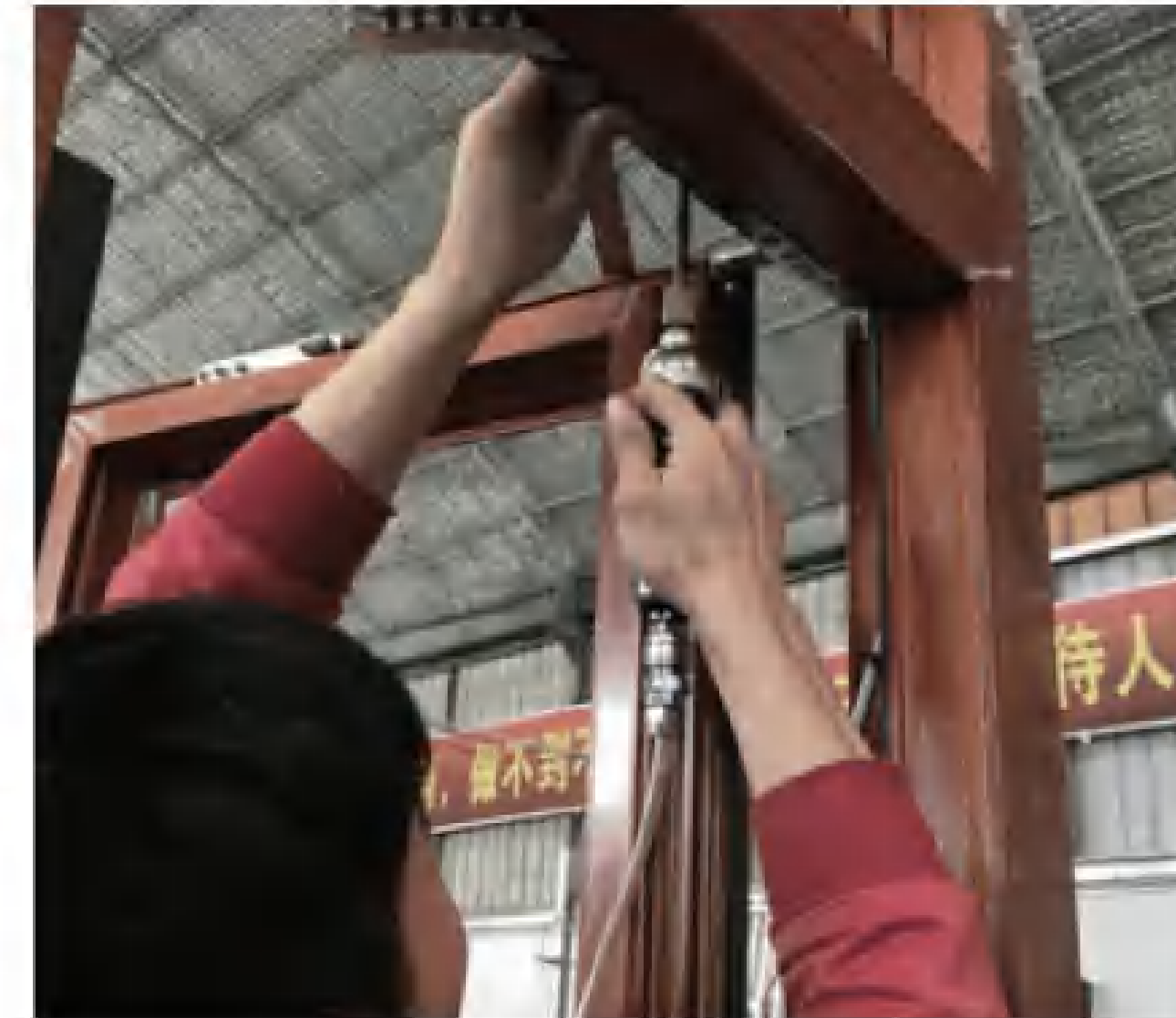
门窗维修 Doors and Windows maintenance
