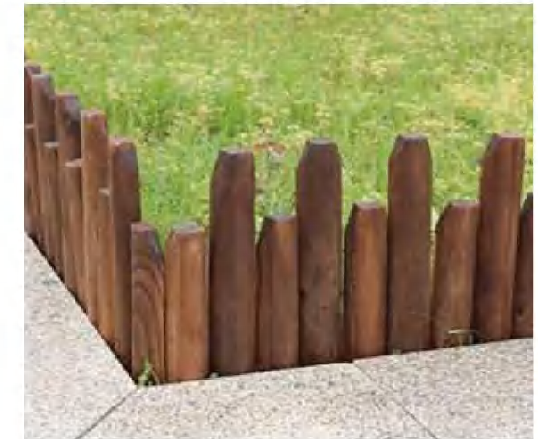
篱笆固定 Fixed the fence
