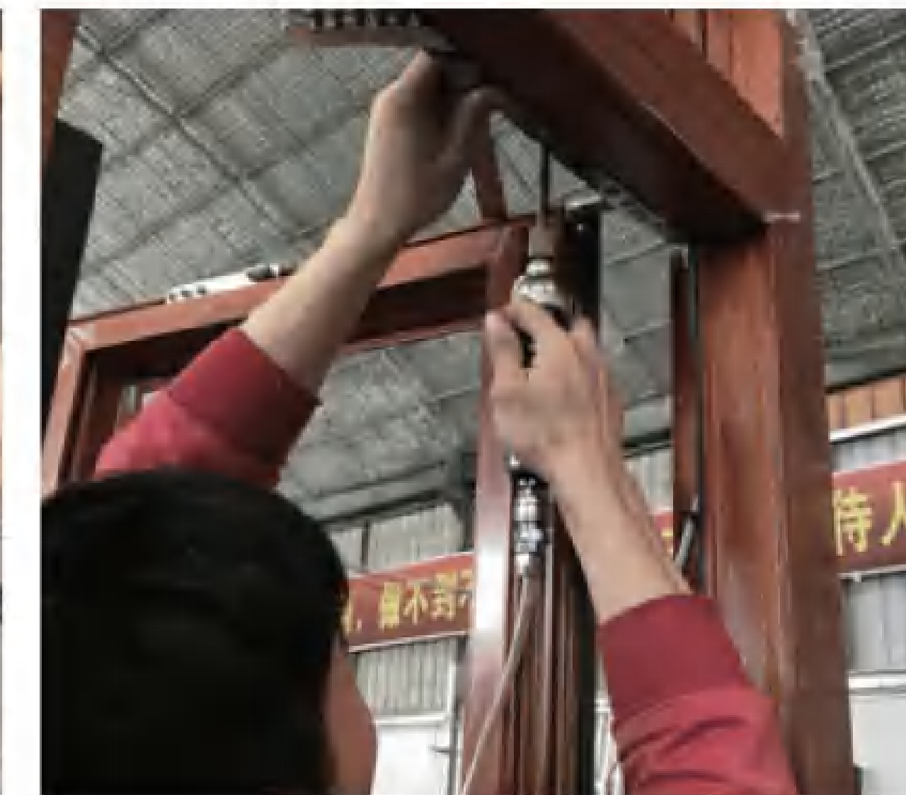
门窗维修 Doors and Windows maintenance
