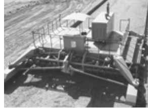
Beton Finiřeri Concrete Finisher
