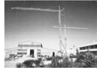
Kule Vinç Tower Crane
